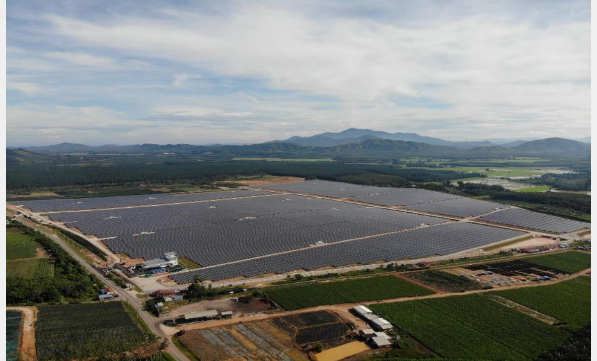
The 65 MW Gurun solar plant in Malaysia.
