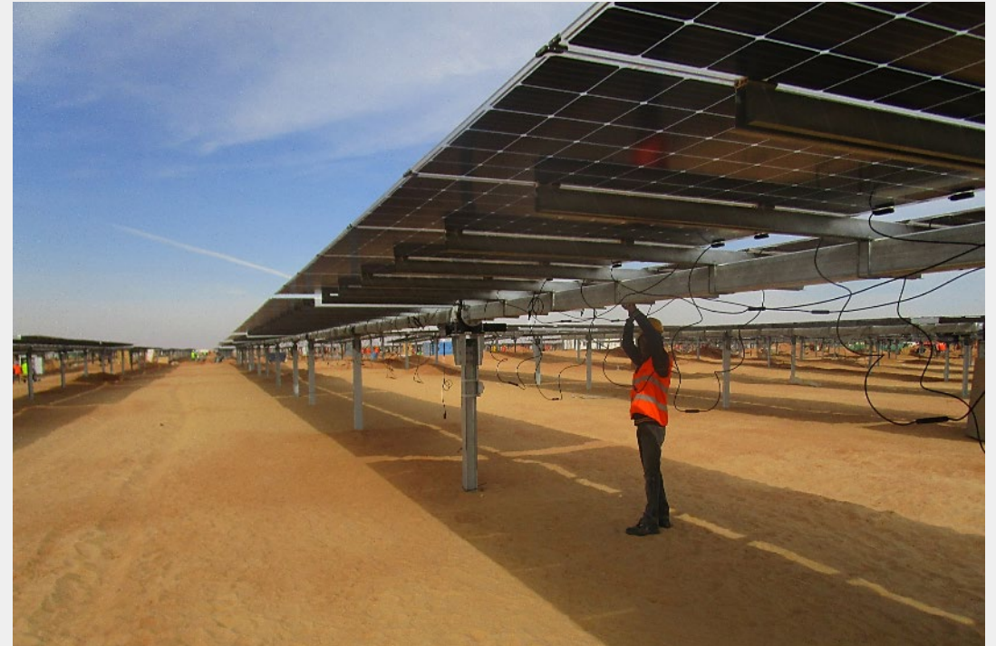
Installation of bi-facial solar panels at the 400 MW project in Egypt.
