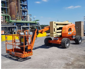
Tertre reduced use of scaffolding on site by 80%
