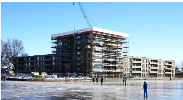
Nieuw Heerenhage in Heerenveen (NL) Development project in progress
