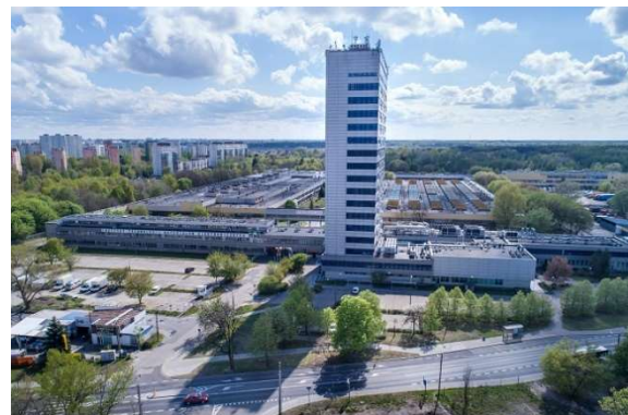
Photo: CeMat complex, Wólczyńska 133, Warsaw, Poland
