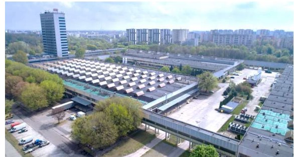
Photo: CeMat complex, Wólczyńska 133, Warsaw, Poland
