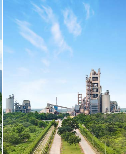
Sagar Cements | Mattampally - Telangana
