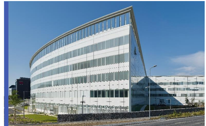
Baikal building, delivered in 2018
