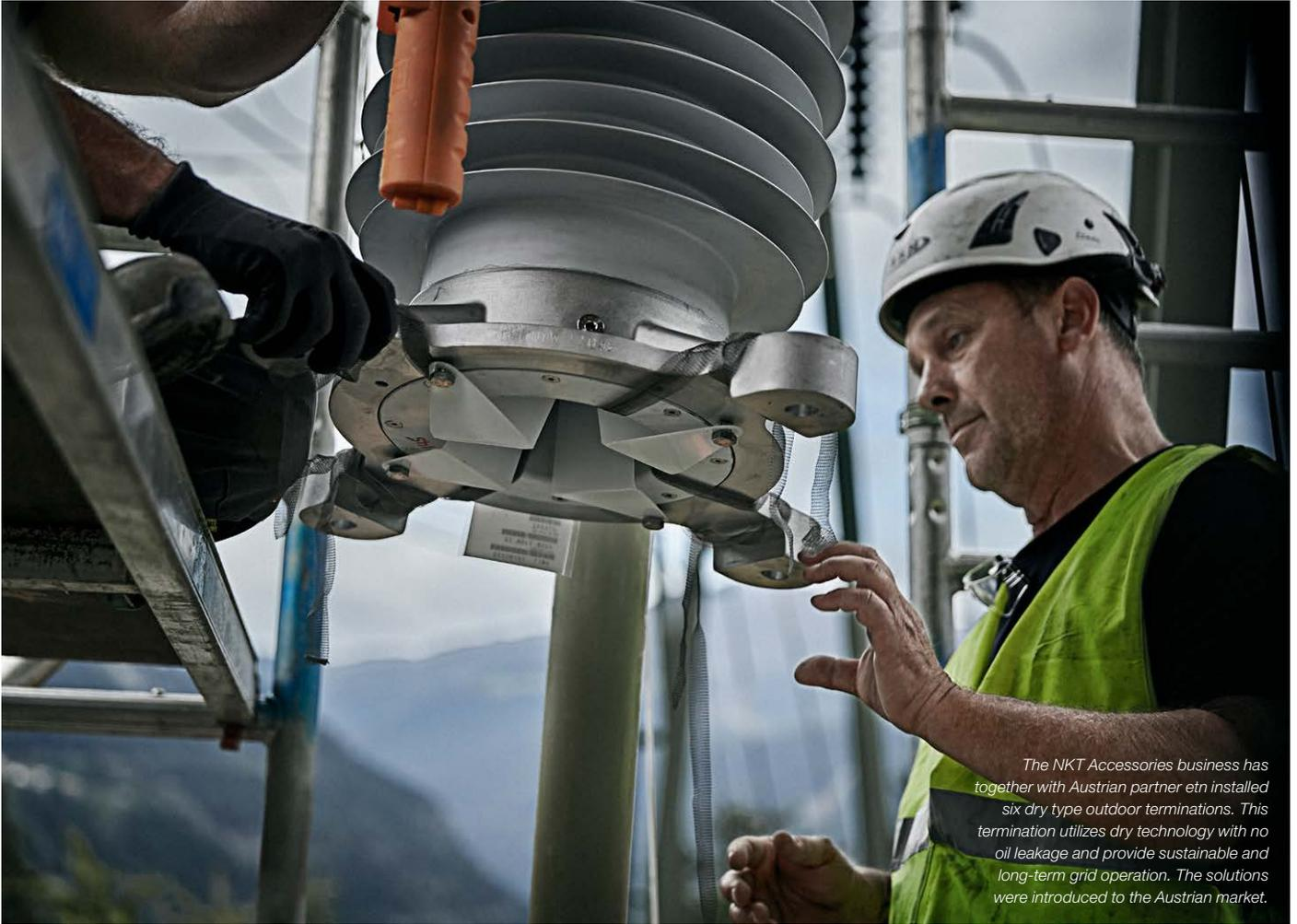
*The NKT Accessories business has together with Austrian partner etn installed six dry type outdoor terminations. This termination utilizes dry technology with no oil leakage and provide sustainable and long-term grid operation. The solutions were introduced to the Austrian market.*
