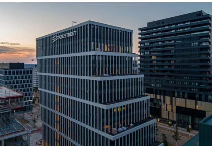
Nextensa • Stairs building at Cloche d'Or, Luxembourg
