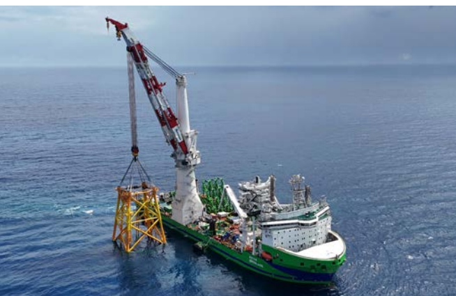
DEME • Installation vessel Green Jade at Fengmiao offshore wind farm in Taiwan
