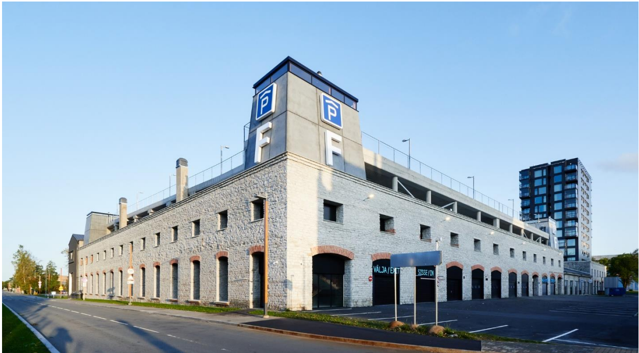
Multi-storey car park at Sepise 8 (Nordecon Betoon OÜ)
