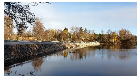
Basic road no. 69, the section between Soontaga and Kuigatsi intersection (Nordecon AS)
