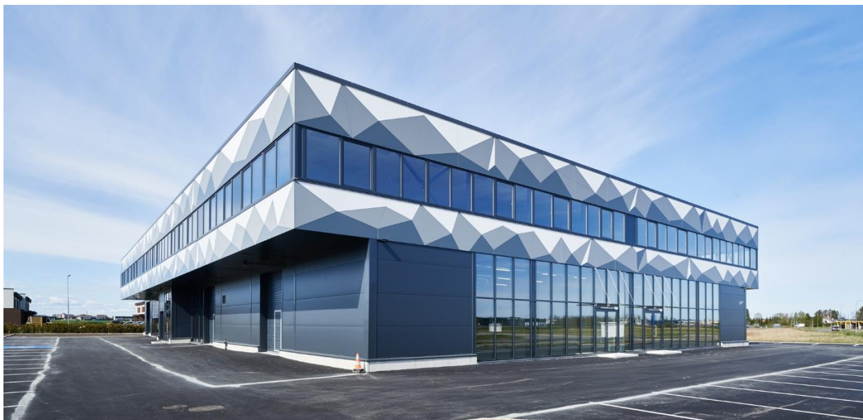
Commercial building at Allika 7 (Nordecon Betoon OÜ)
