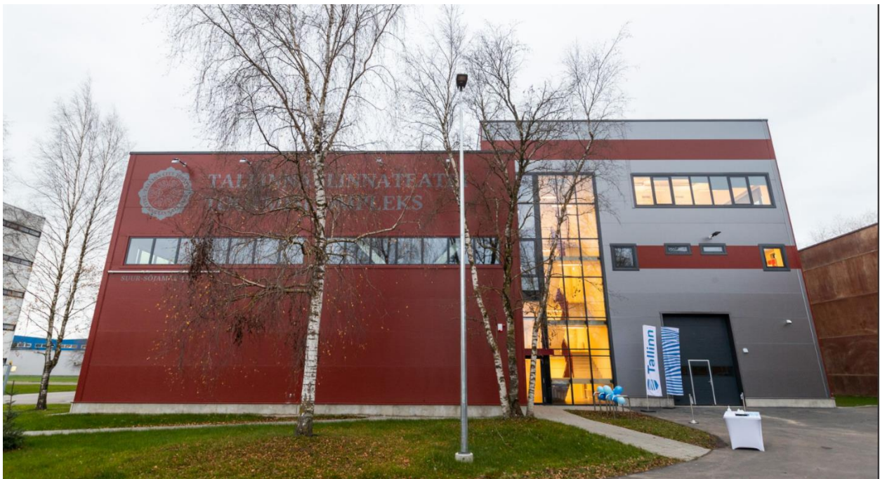
Production complex of Tallinn City Theatre (Eston Ehitus AS)
