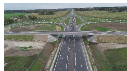
National road no. 4 (E67), Kernu bypass (Nordecon AS)
