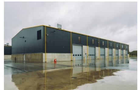
Maintenance and training facility in Tapa (Nordecon AS)
