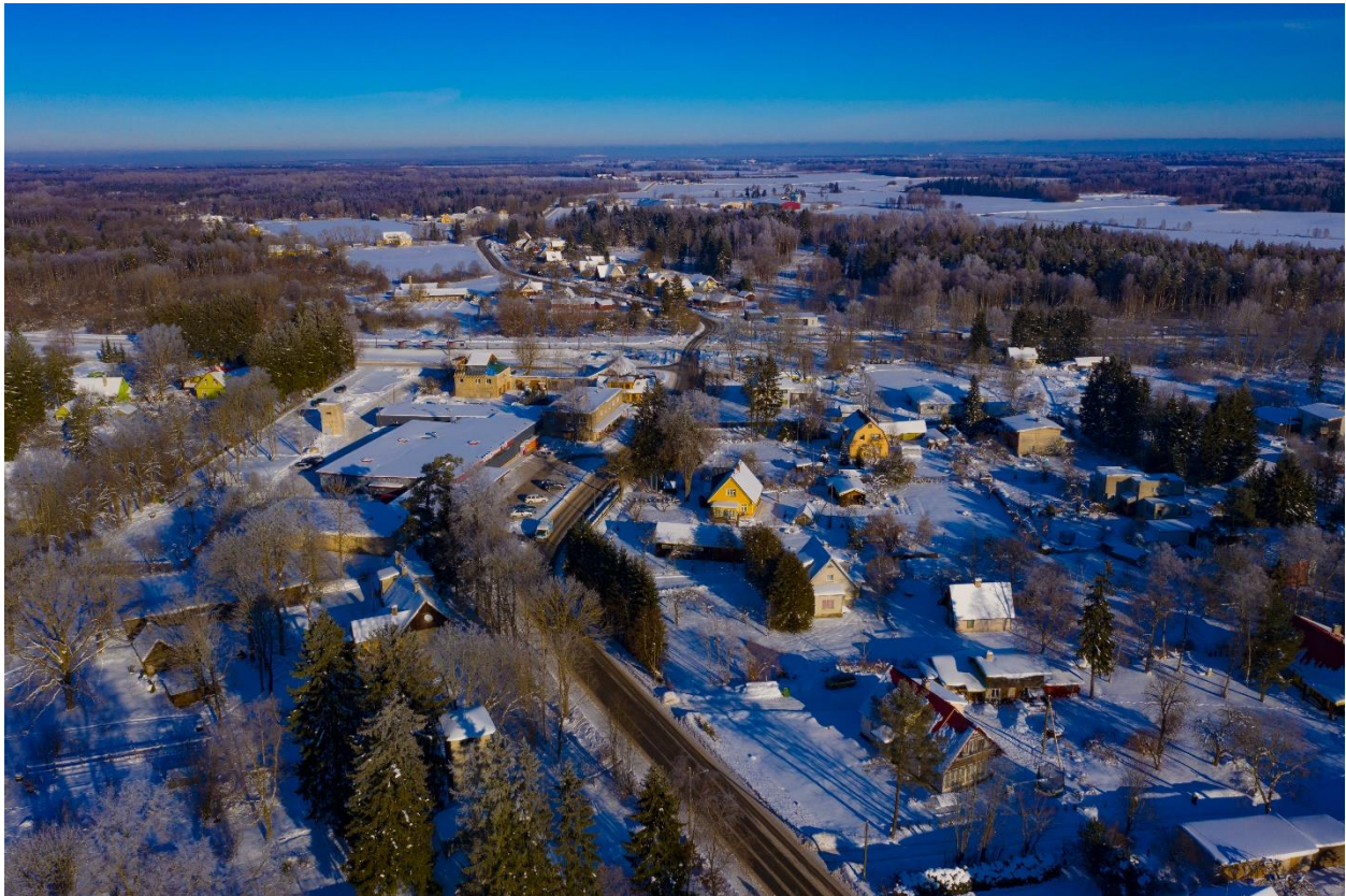
Aruküla-Kostivere road section (Nordecon AS)
