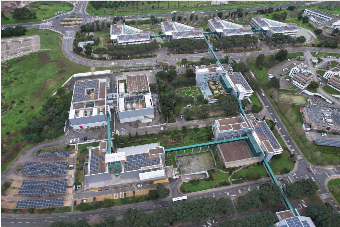
2 nd photovoltaic plant - central services in Taguspark (Portugal)
