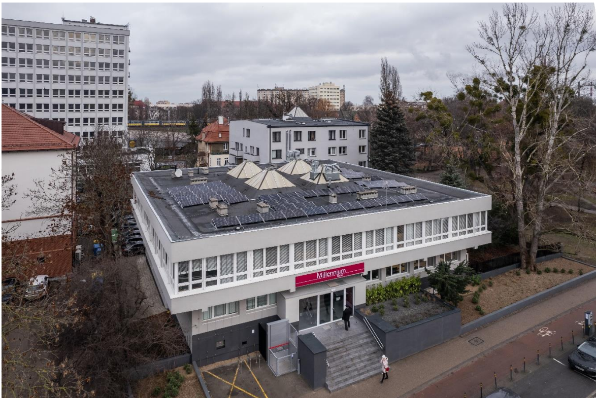
Photovoltaic plant - central services in Gdansk (Poland)
