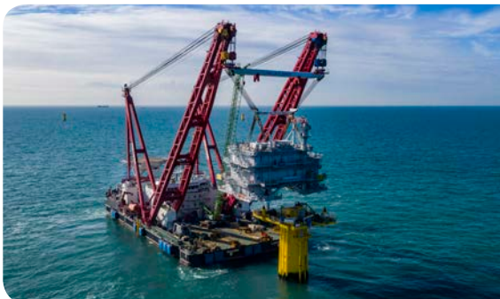
DEME - SeaMade - Installatie van offshore substation
