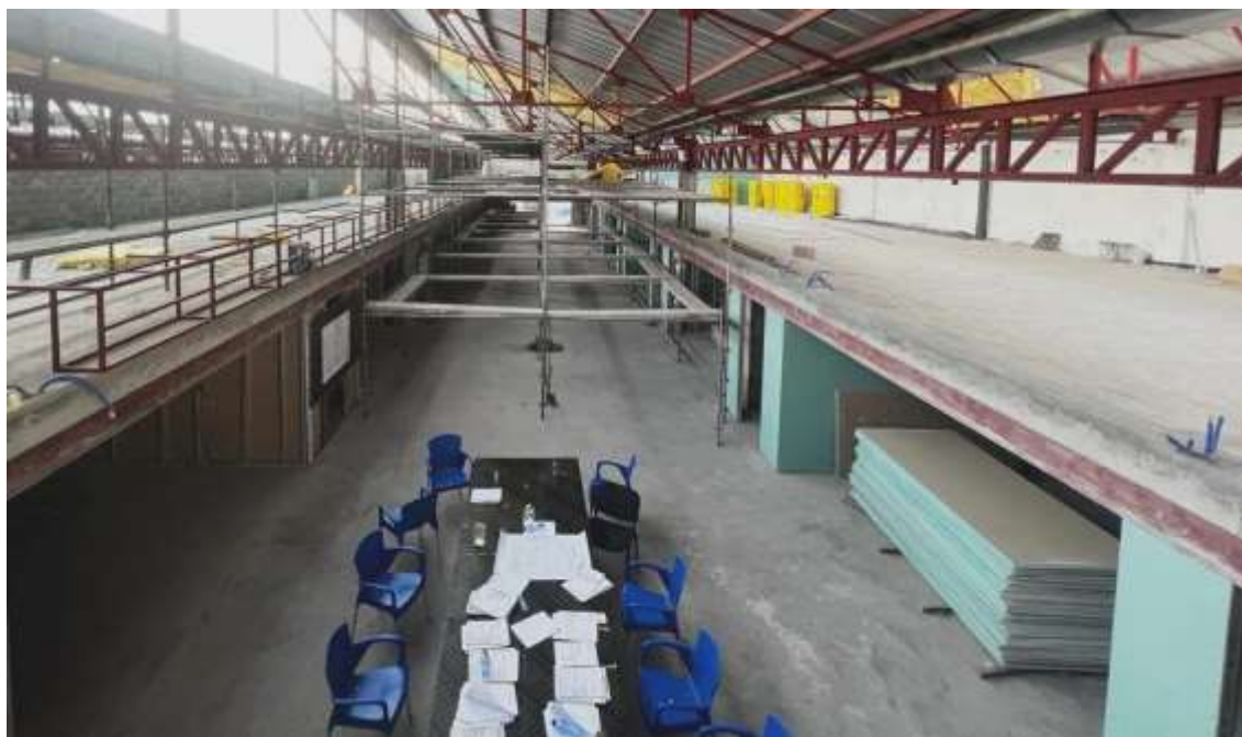
Chantier Silikin Village III
