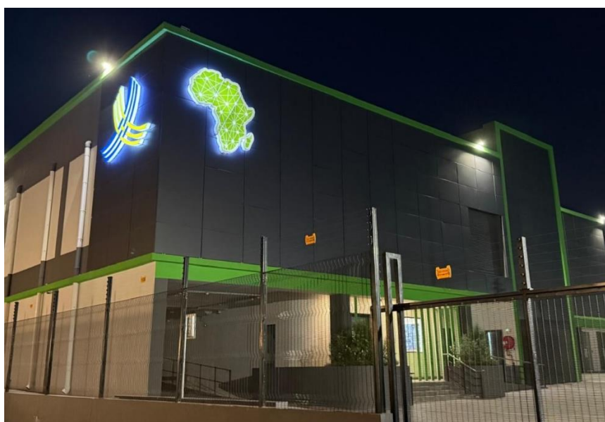
Data centre OADC Texaf Digital
