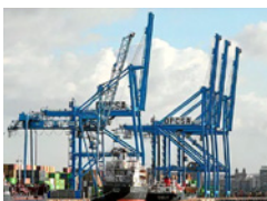
OPCSA has JLT rugged computers installed in all ship-to-shore cranes, rubber tire gantry cranes, reach stackers, and prime movers.
