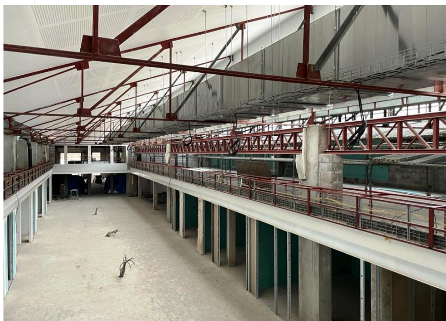
Silikin Village Phase III construction site
