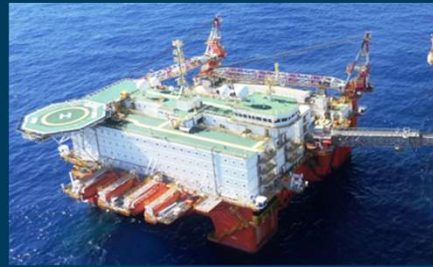
Safe Notos – Petrobras 2030 Built 2016 – 500 beds
