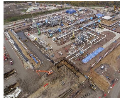
Nord Stream 2 onshore facility
