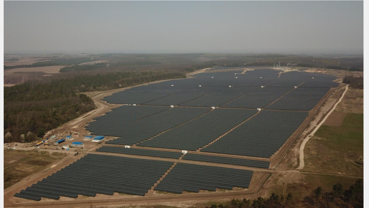
The 54 MW Boguslav solar plant, Ukraine.
