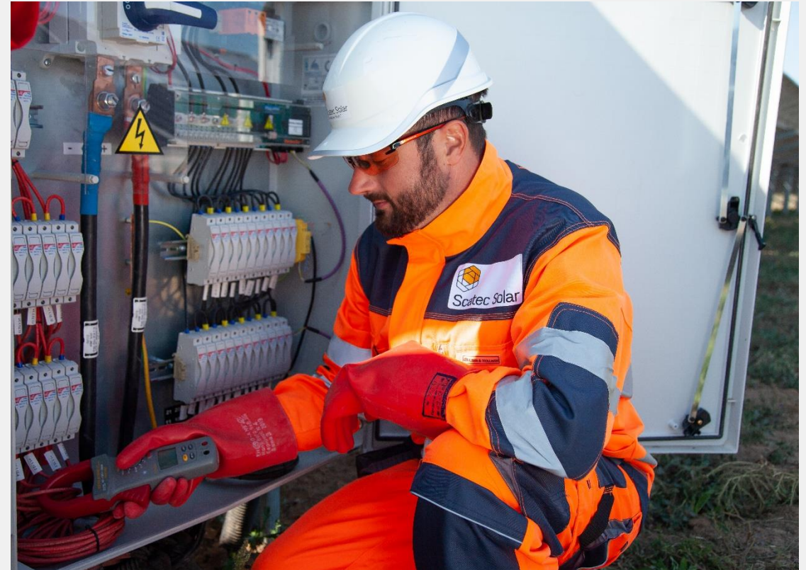
Installation work ongoing in Ukraine.
