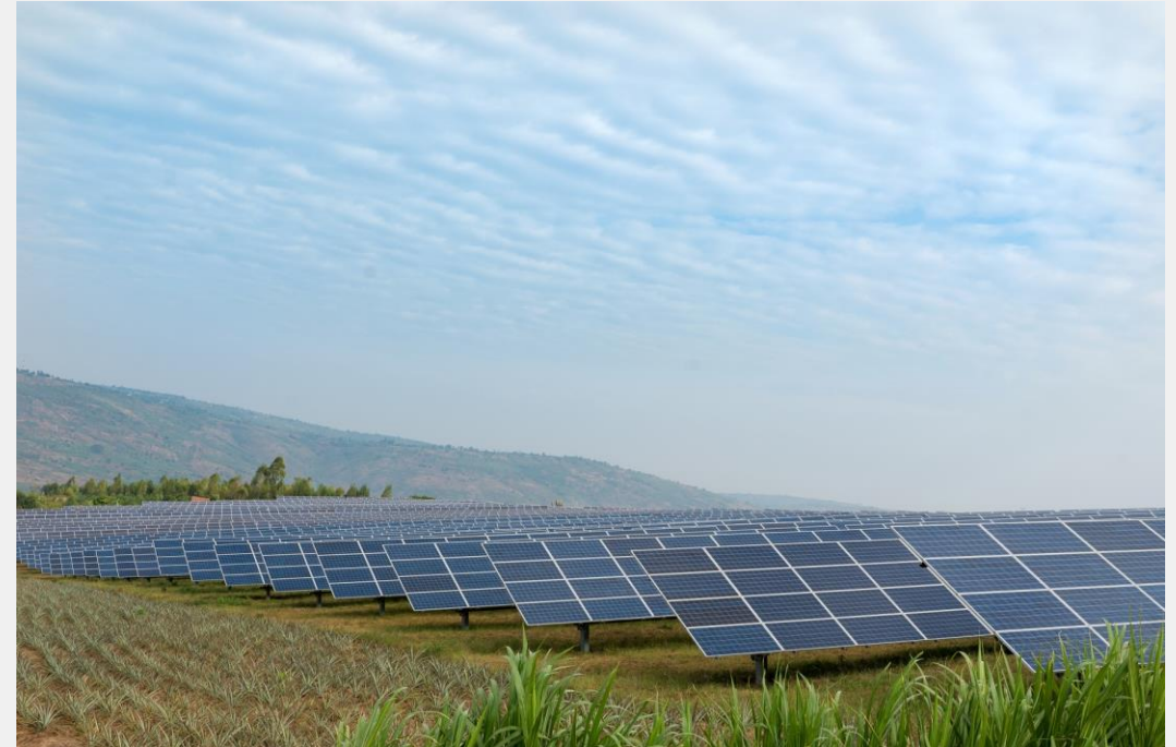
The 9 MW Asyv plant, Rwanda.
